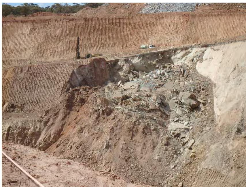
Figure 3.36 Wattlebird open pit wall failure
