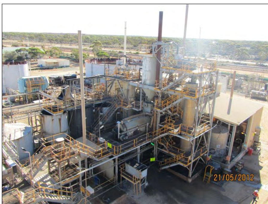
Figure 3.47 Elution and carbon regeneration circuits
