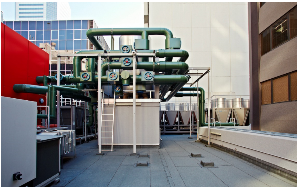
Air-cooled UNIFLAIR chillers and water storage (B1)
