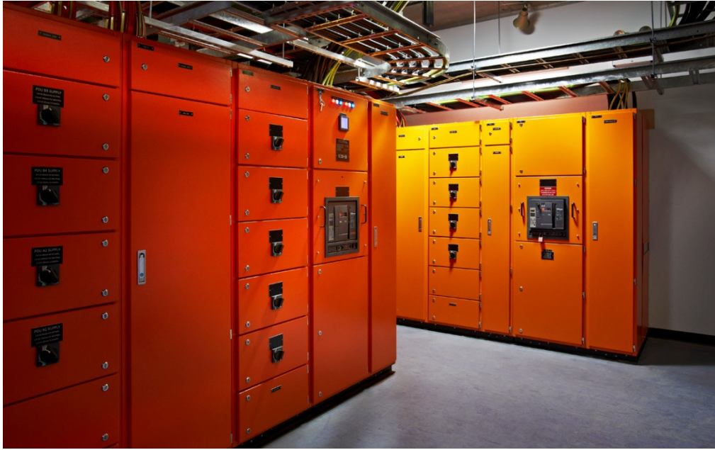
High Voltage switchboard (C1)
