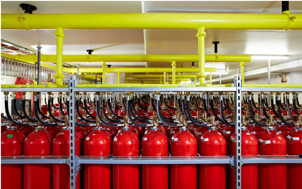
Inert gas fire suppression system (S1)
