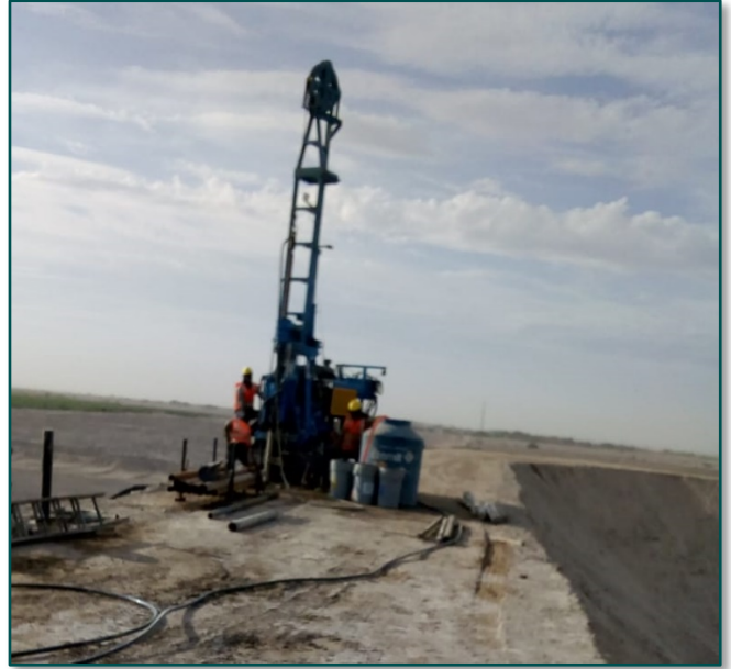
Figure 3 | Drilling of water monitoring wells in accordance with environmental management plans at the Vista Tailing Dam.
