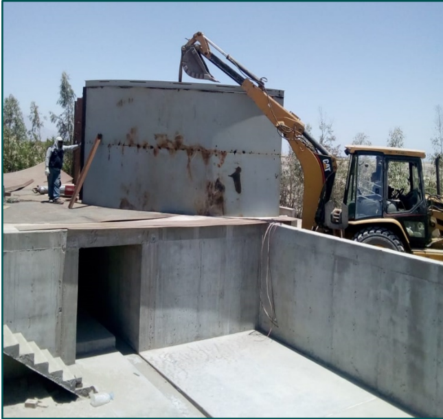
Figure 2 | Installation of Tailing Thickener.
