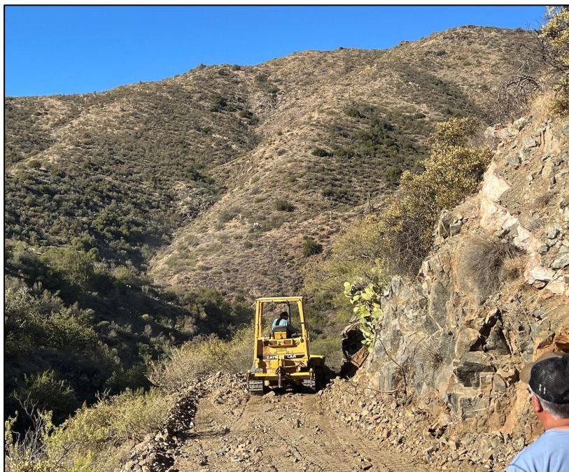
Photo 1 – Earthworks in progress to establish drill pads aimed at testing porphyry-style targets.
