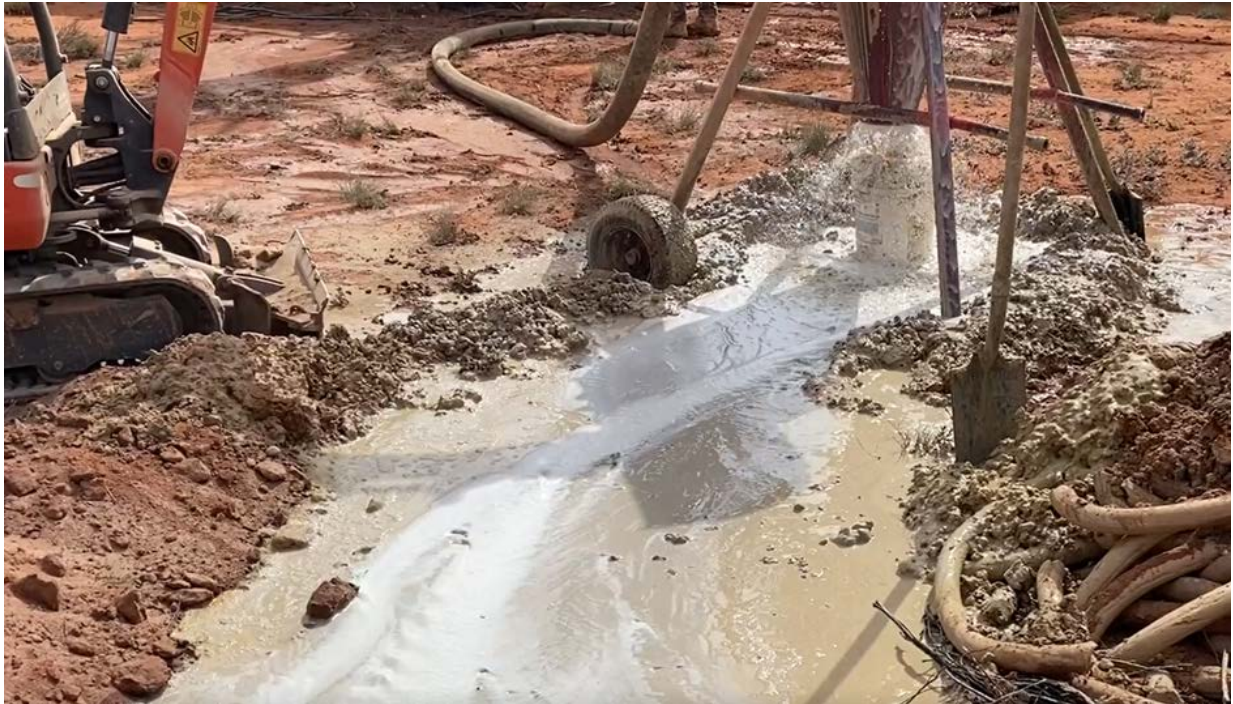
Figure 6. Brine flowing from cyclone at 78m from LWP002
