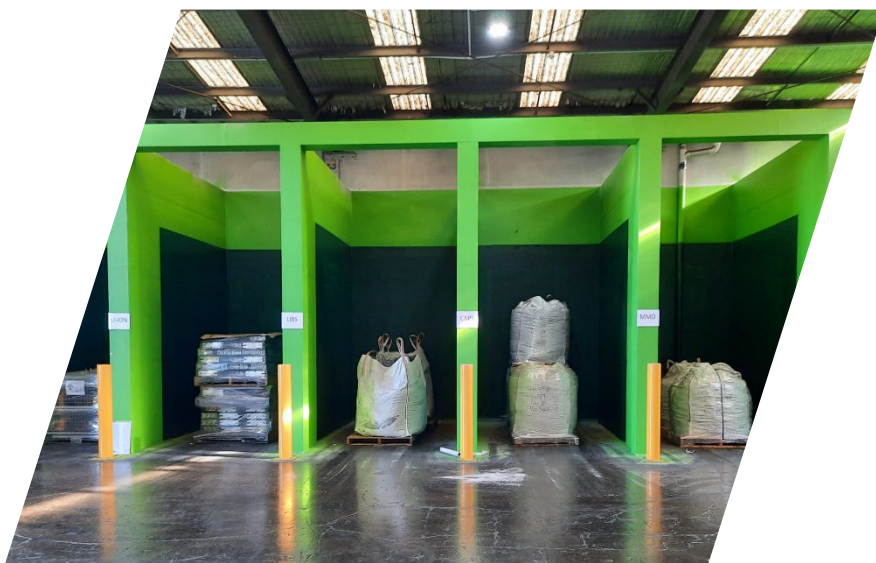
Top: Fireproof box, Bottom: Firewalls at Berwick Road facility
