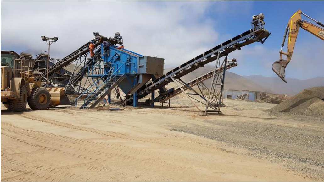
Tertiary circuit vibrating screen being installed mid November
