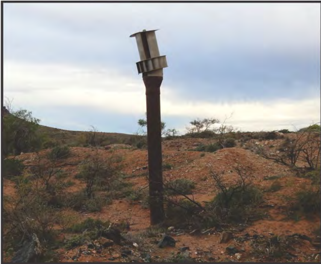
Photo 3-5: Small Vent Shaft Source: ERM
