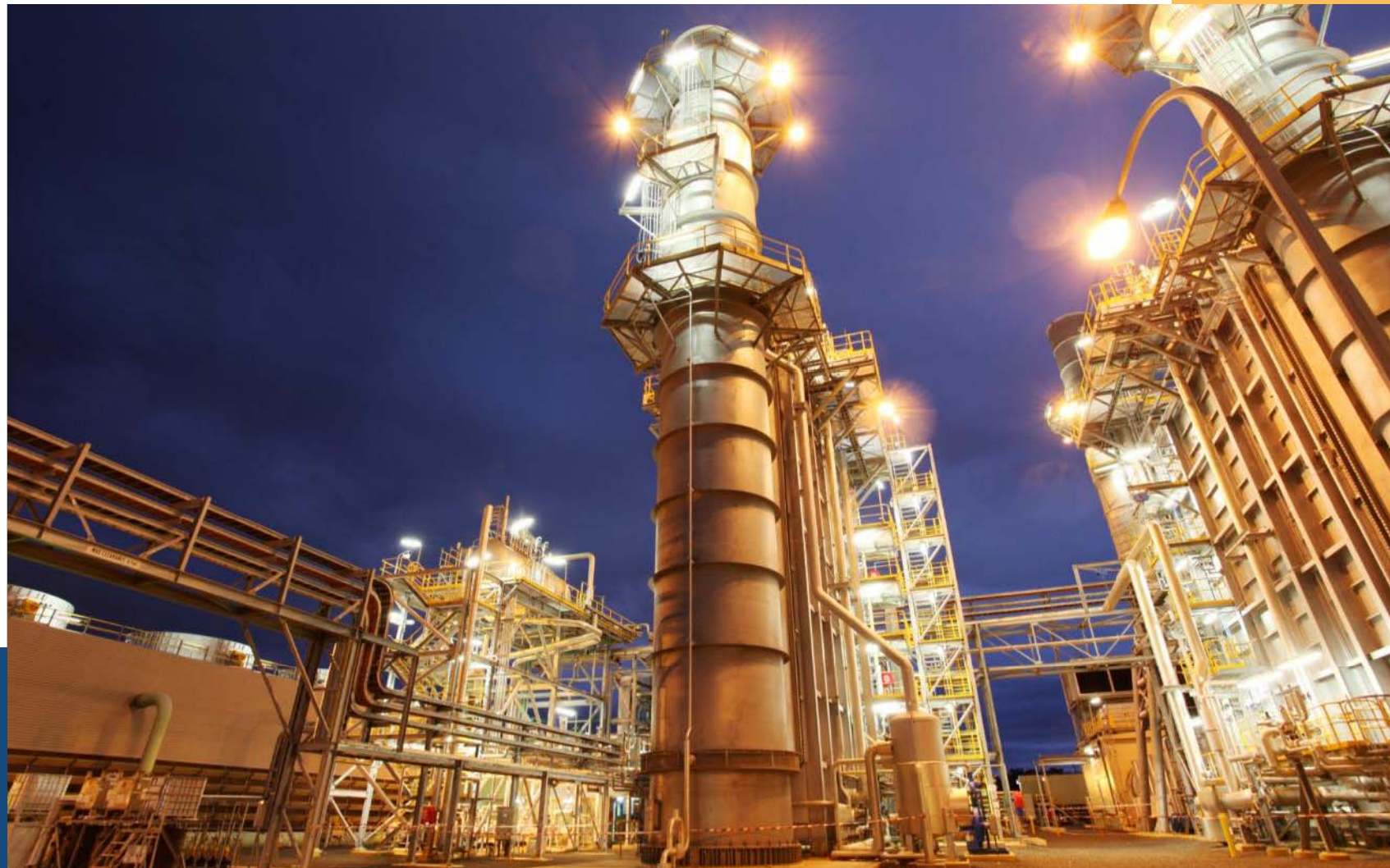
Completed Heat Recovery Steam Generators ("HRSGs") using RCR proprietary technology, QLD
