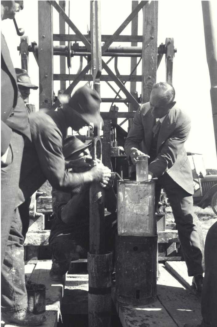
Gas sampling whilst drilling – Ramsay Oil Bore
