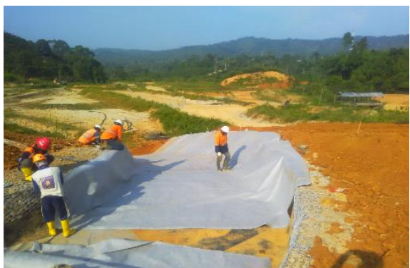
Construction of Talang Santo Pit Spillway
