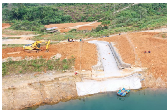
Construction of Talang Santo Pit Spillway
