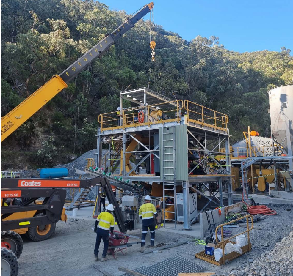
Figure 9 Ore sorter installation well underway
