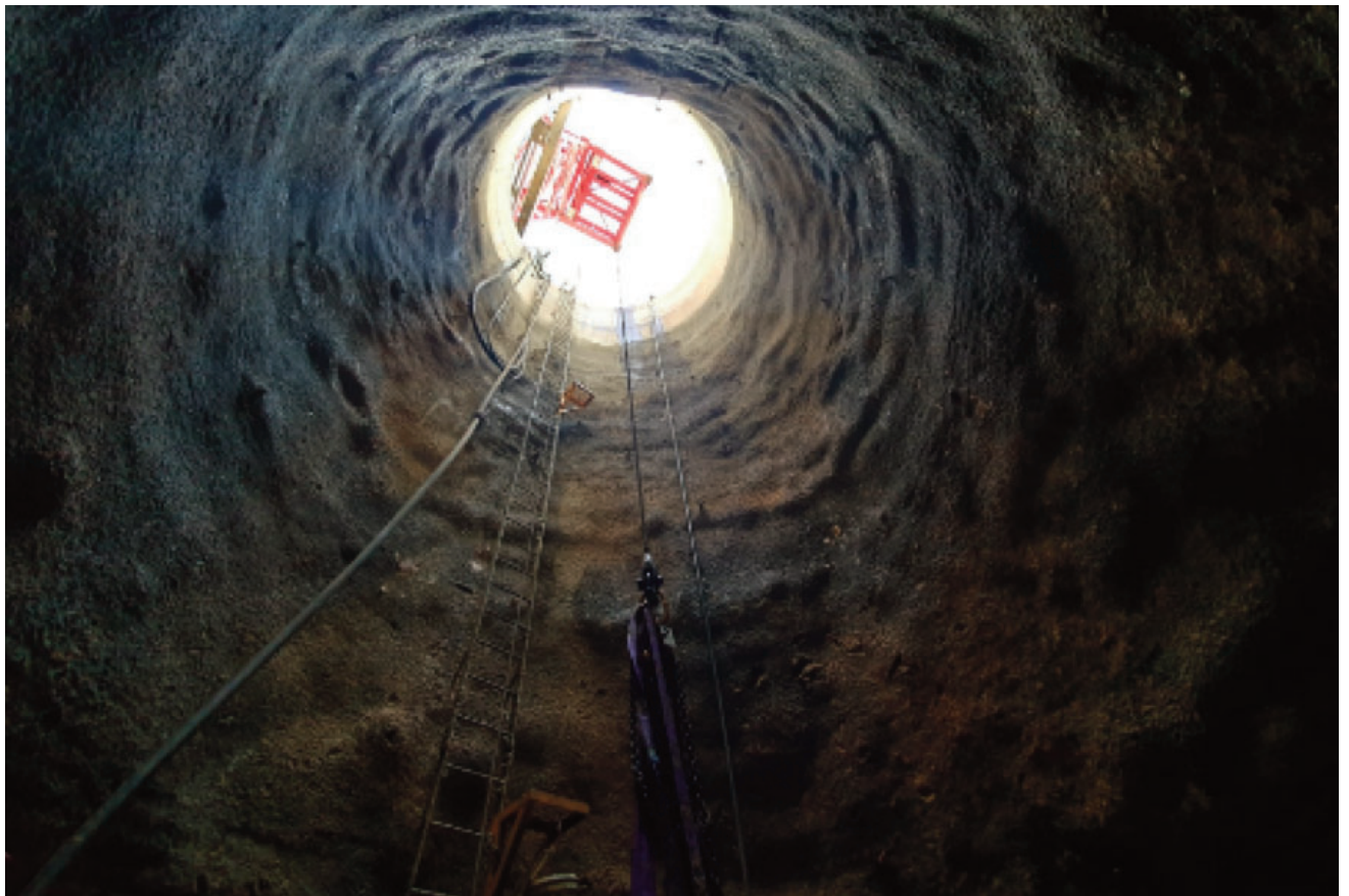
Figure 10: Woodlawn primary ventilation shaft.
