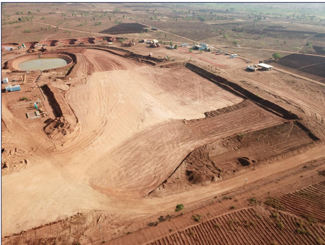
Figures 3 & 4: Test pit during hydro-mining trials (above) and aerial view of test pit being backfilled
