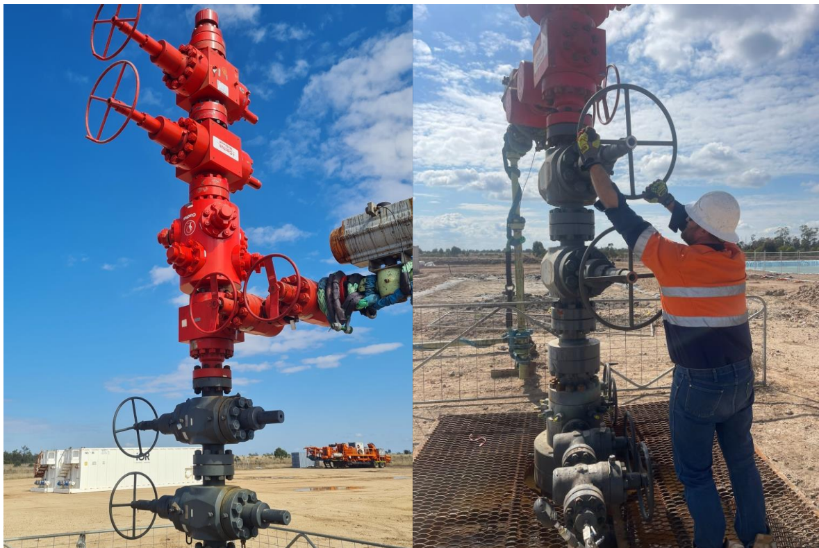
Servicing of well head at Daydream-2
