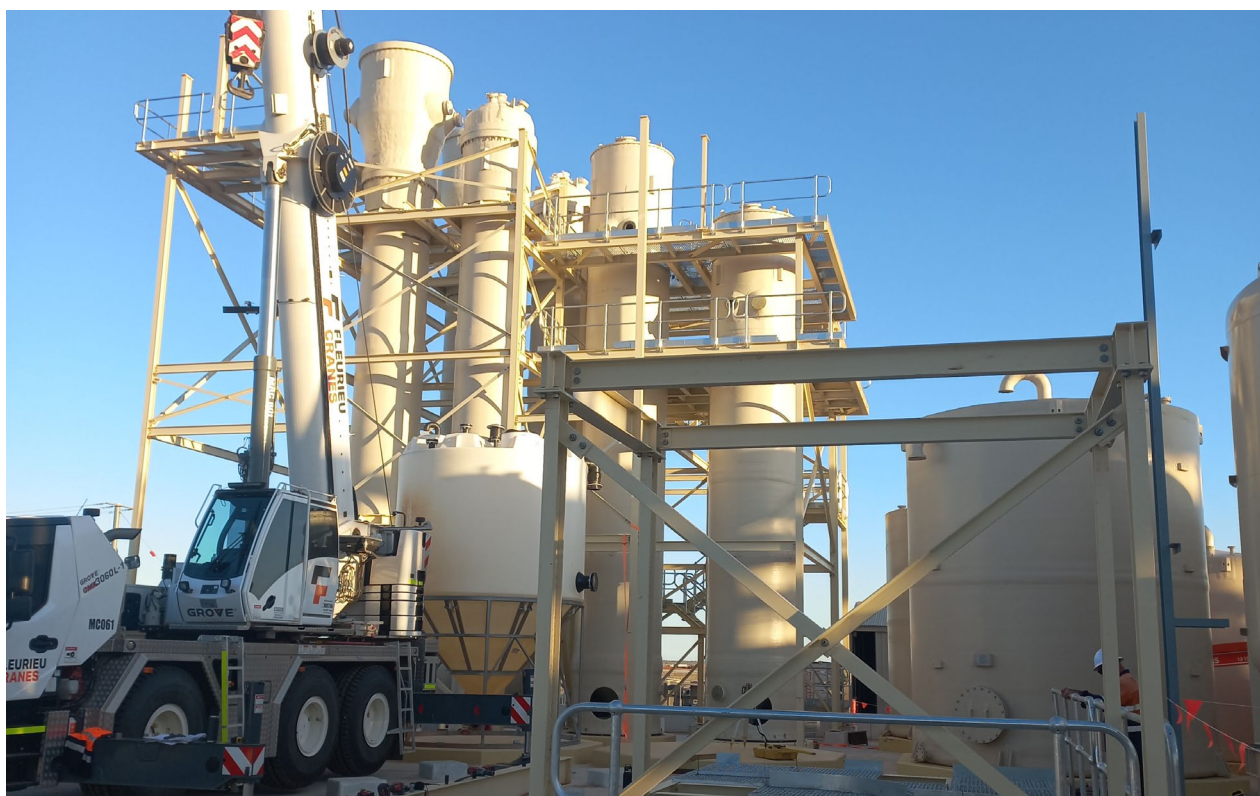
Installation of ion exchange columns for Heathgate Uranium Processing Plant, South Australia
