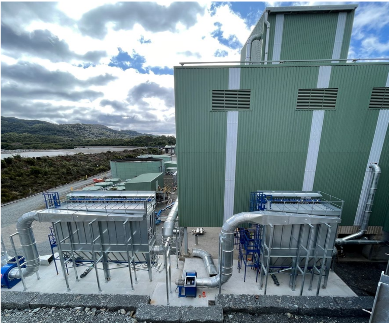
Figure 4. Dust Extraction System at the Crusher House
