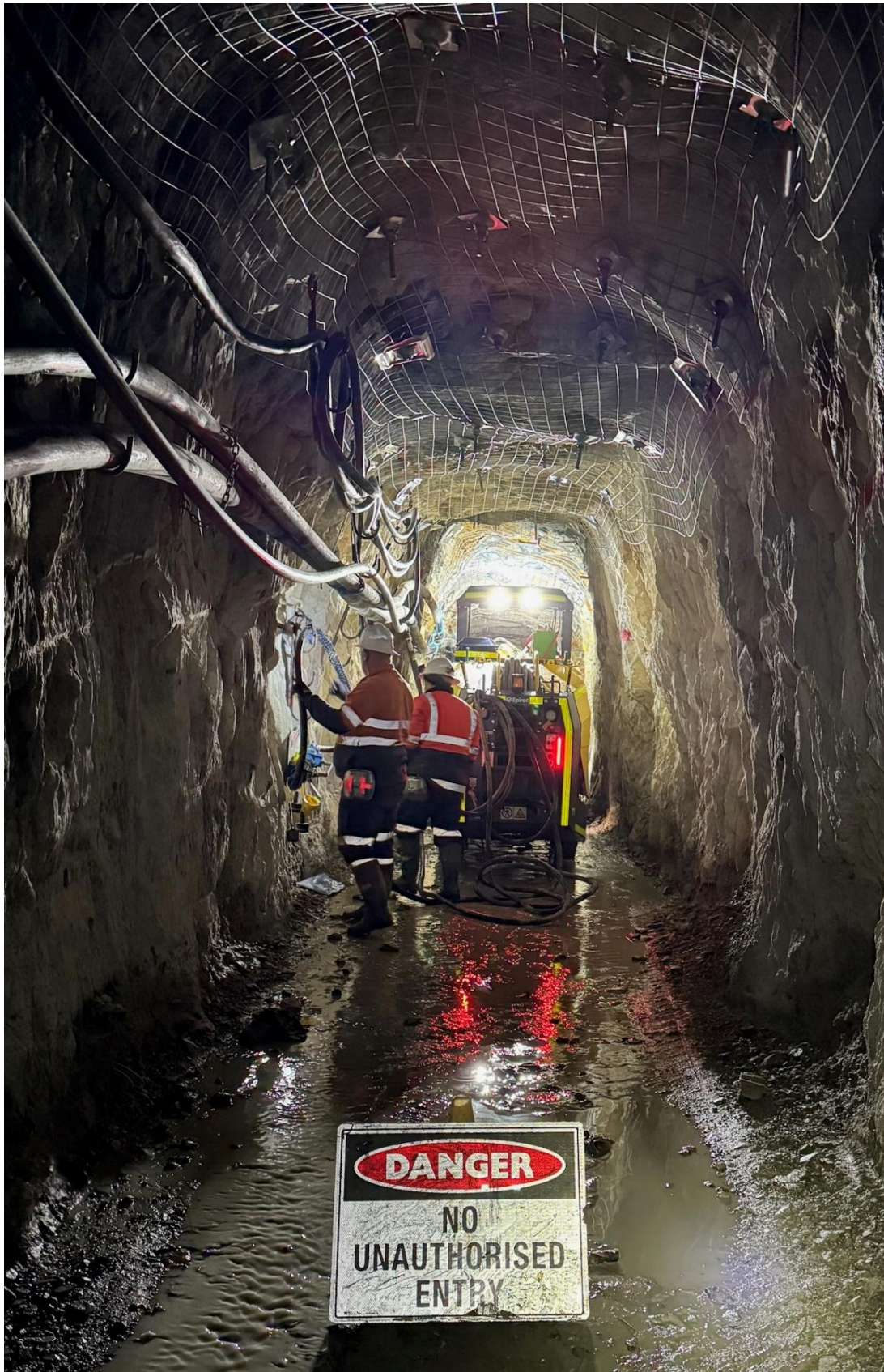
Figure 4. Vertex Mining crew lifting the height of the backs (roof) to enable 11kva cable and other service piping to be hung safely away from the mobile mining equipment.
