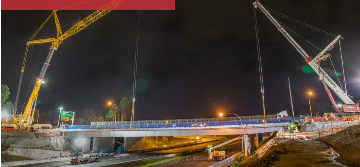
Seymour Whyte successfully installed a 52 m long, 66-tonne bridge girder—the largest in company history
