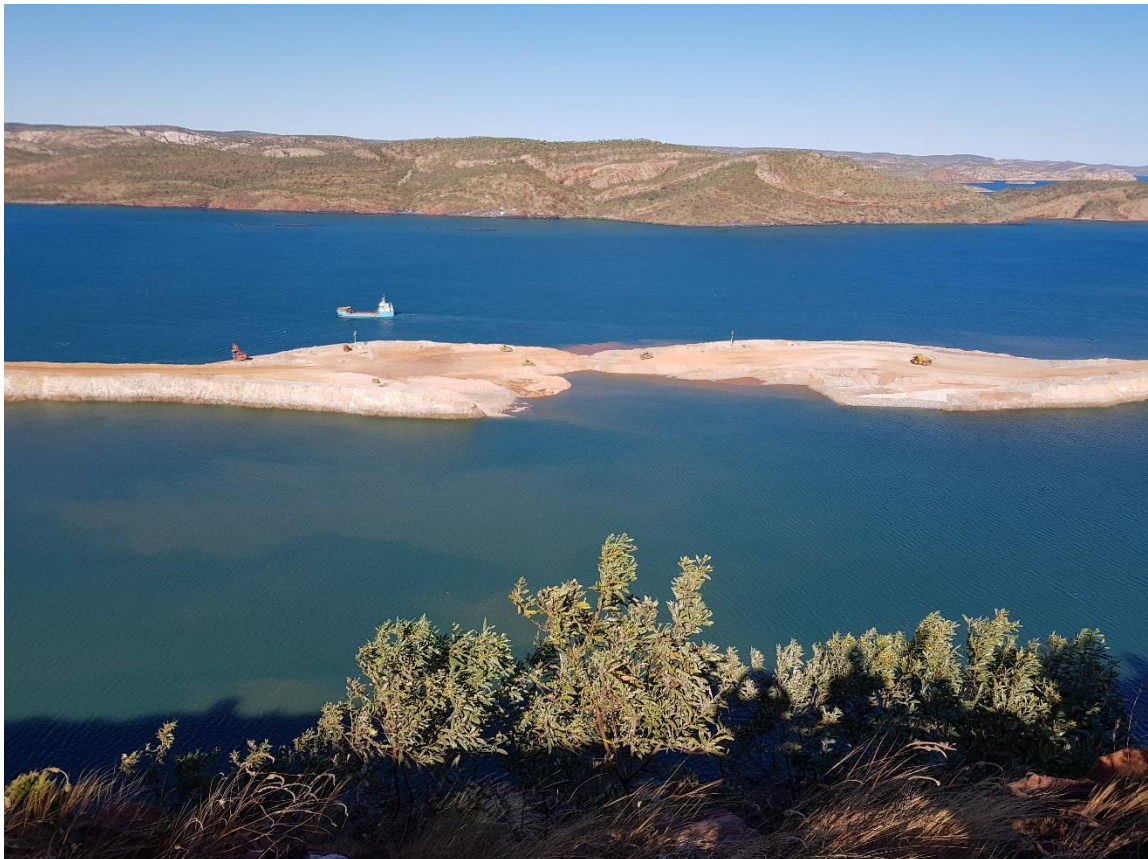
Figure 3: Starter embankment showing closure of seawall breach, 3 August 2017.
