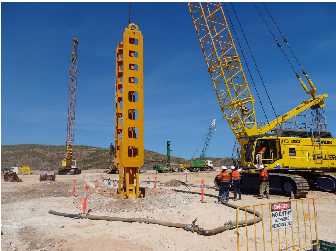
Figure 7: Pilot seepage barrier panel excavation – 28 September 2017
