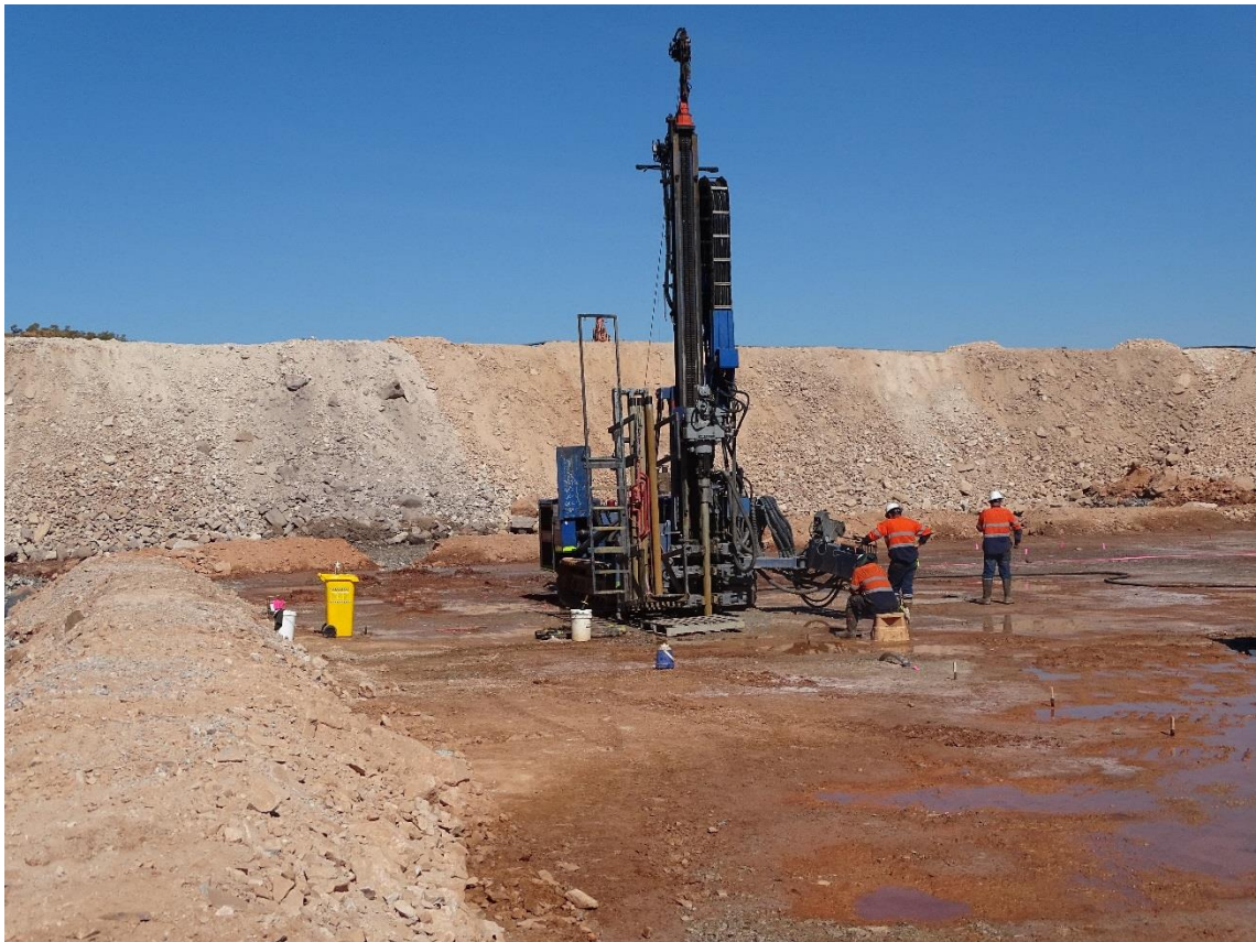
Figure 8: Drilling vertical drains – 29 August 2017
