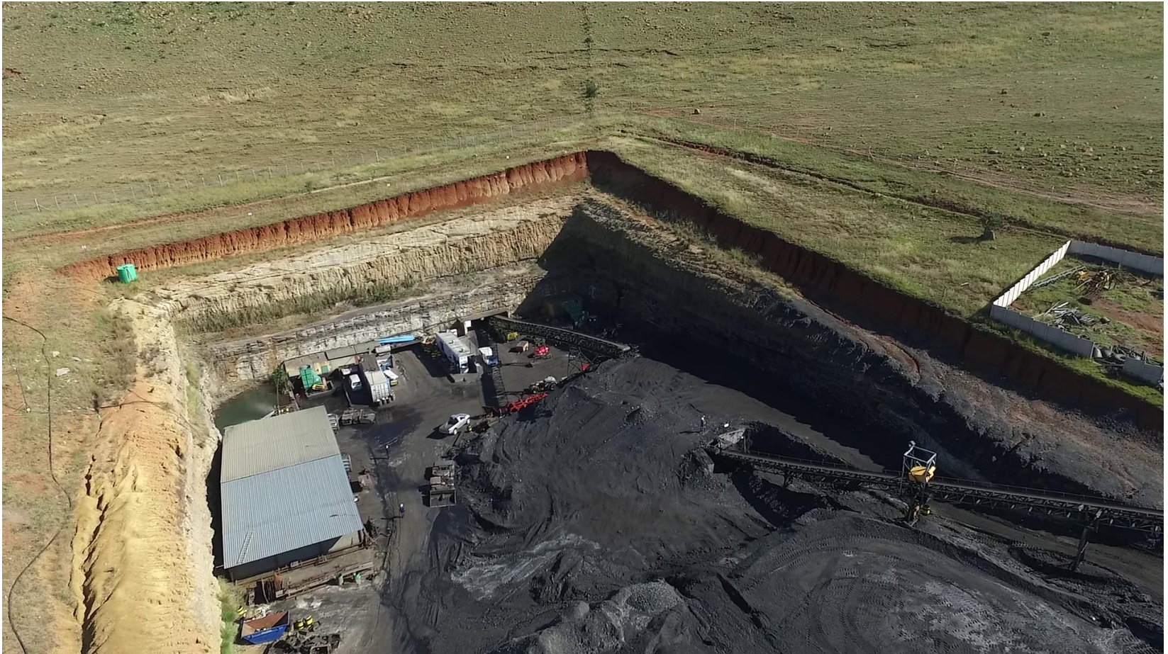
Uitkomst Colliery south adit and conveyor to the processing plant
