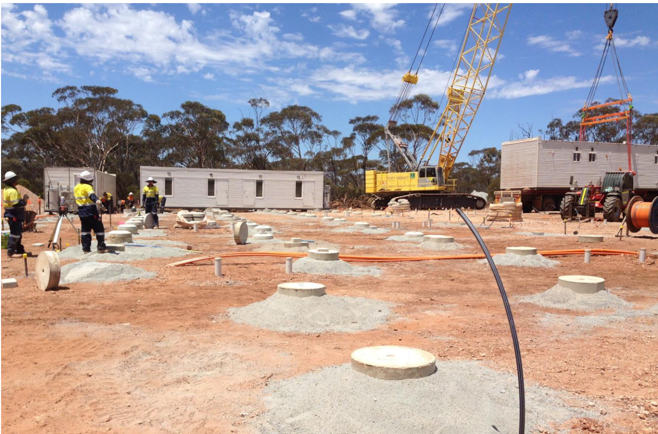
Figure 6. Construction camp expansion - footings for accommodation units
