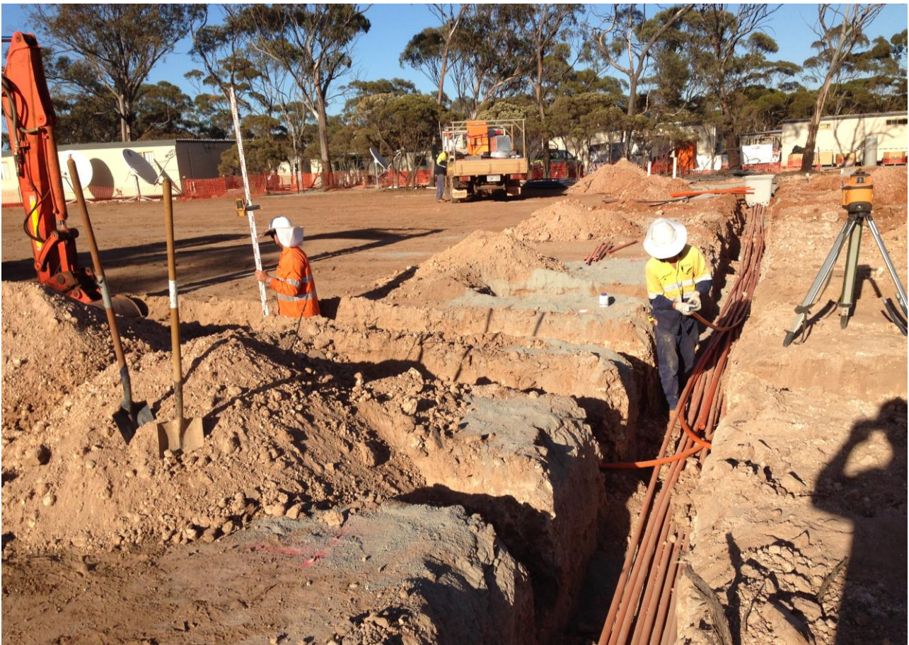
Figure 5. Construction camp expansion – laying underground services
