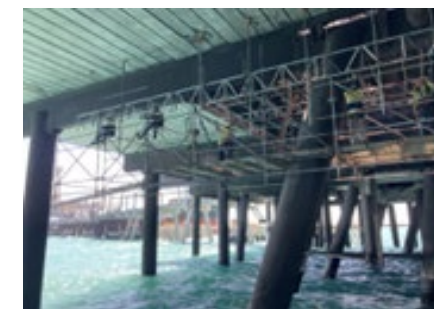
Scaffolding in place for Pile Wrapping Project
