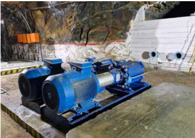
Photo 3: Underground 178m Level Multi-Stage Pumps.
