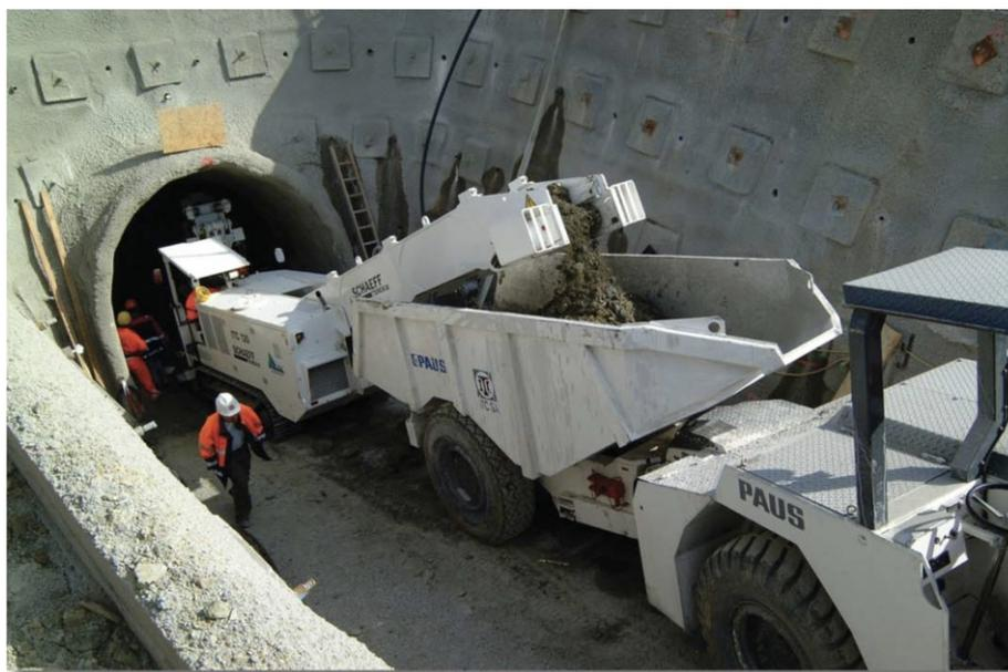
**Photo: ITC Loader and paired Paus bi-directional haul trucks to be used in the trial mining.**
