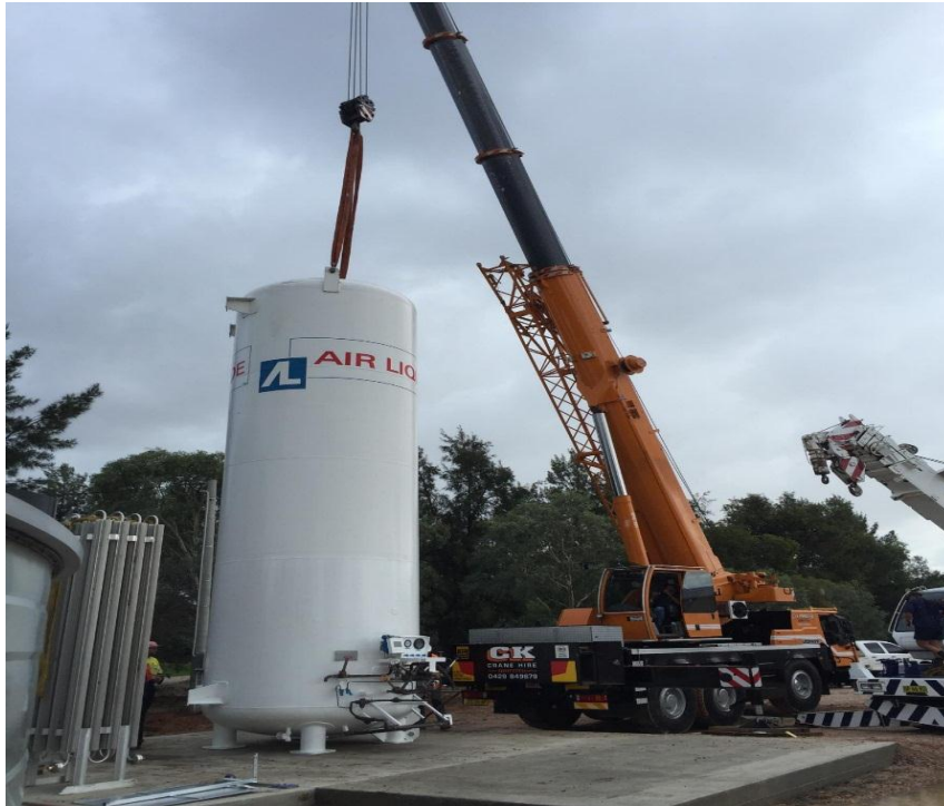
Bulk Oxygen Vessel Being Installed at Bilbul Site
