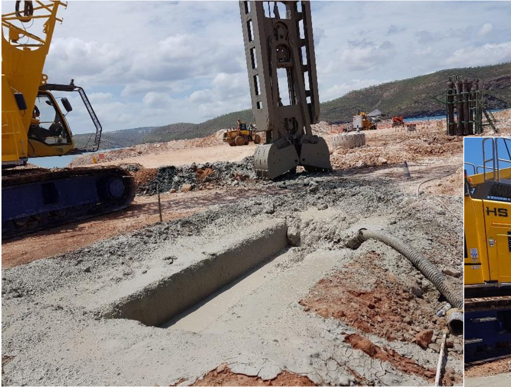
Pumping slurry into excavated Panel 011 December 2017
