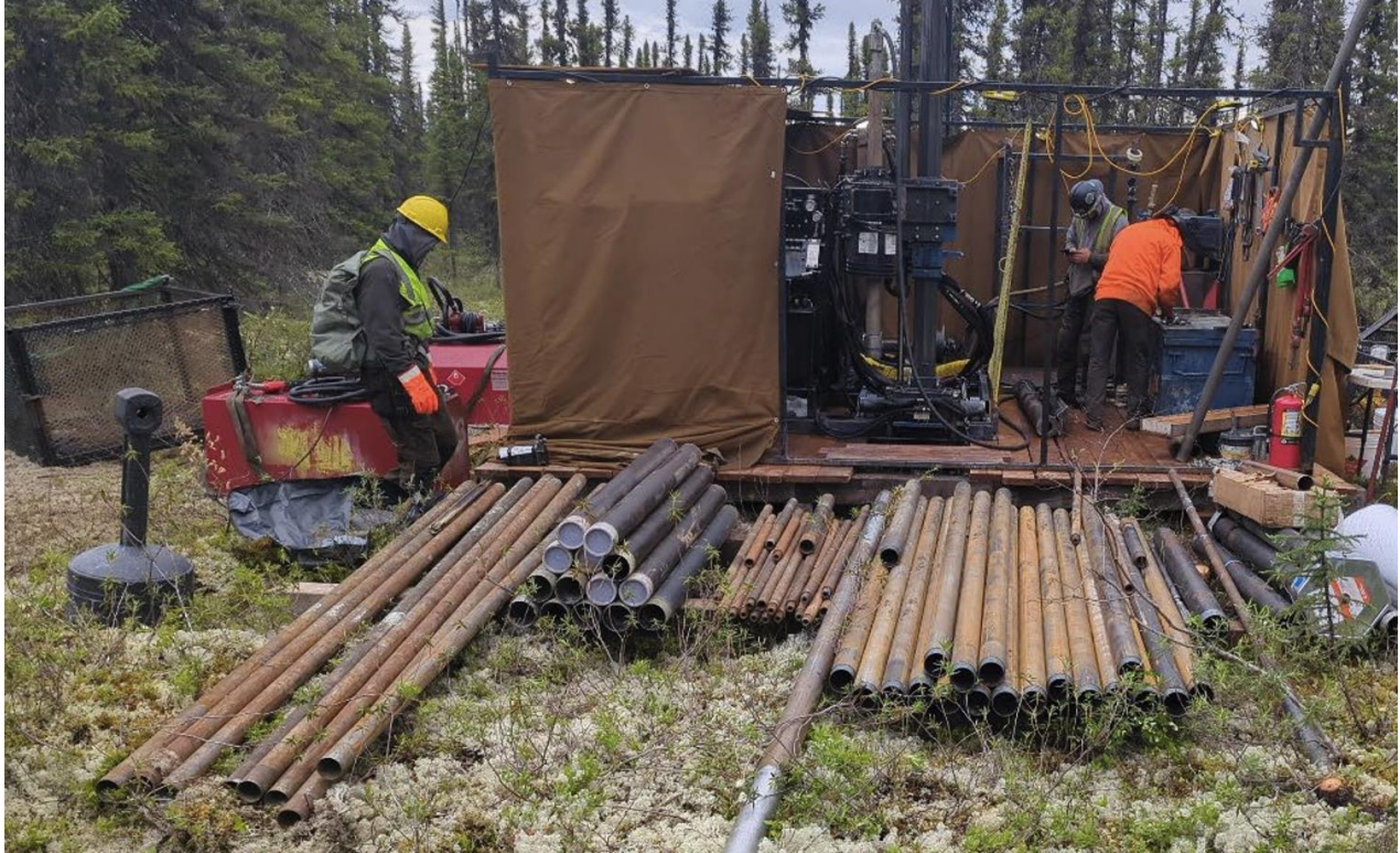
Figure 1: Site of drill hole CV24-537, situated north of CV5, completed for geotechnical purposes and monitoring well installation.
