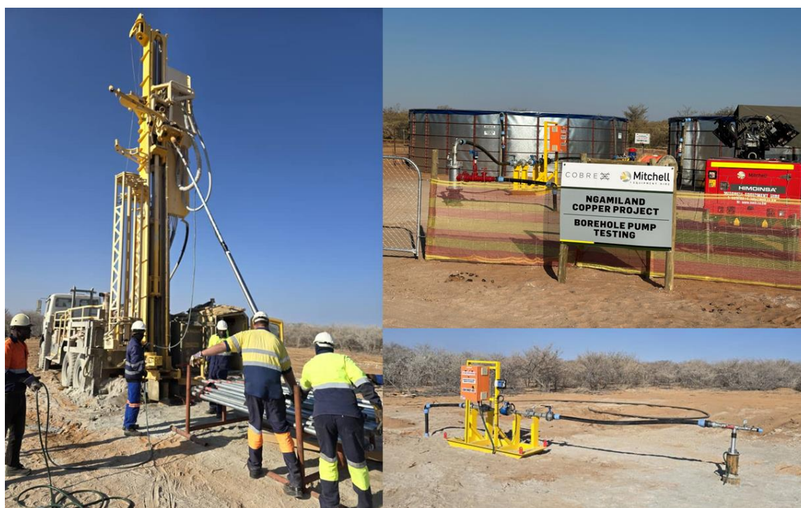
Figure 3. Drilling and development of pumping well PW02.
