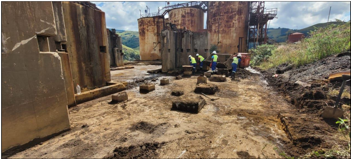
Figure 6: Cleaning of old mill structures in preparation for drilling and blasting
