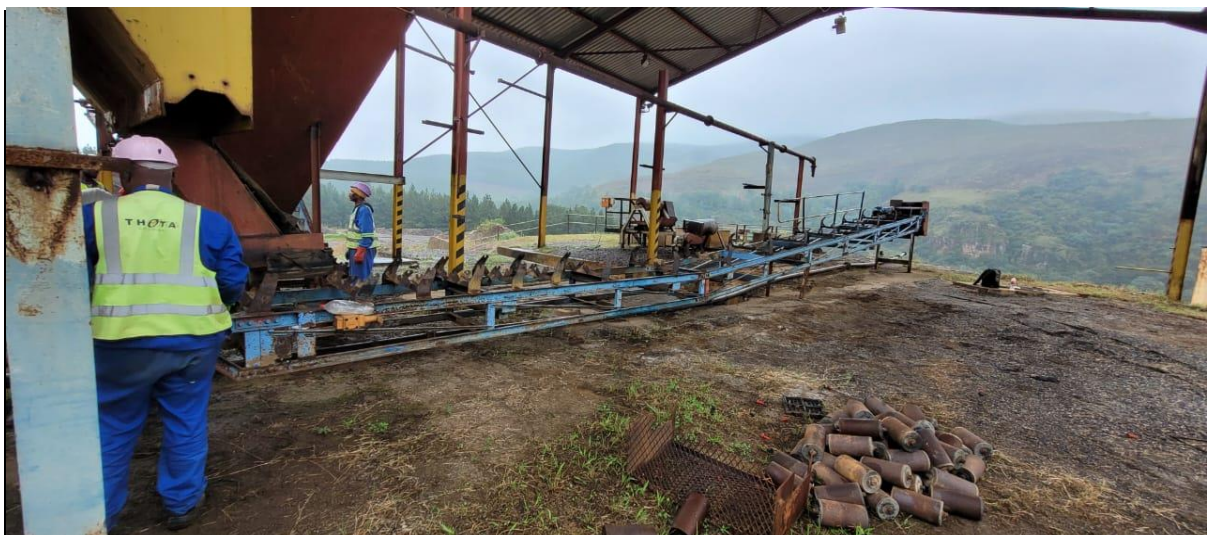
Figure 5: Removal of old conveyor belt structure
