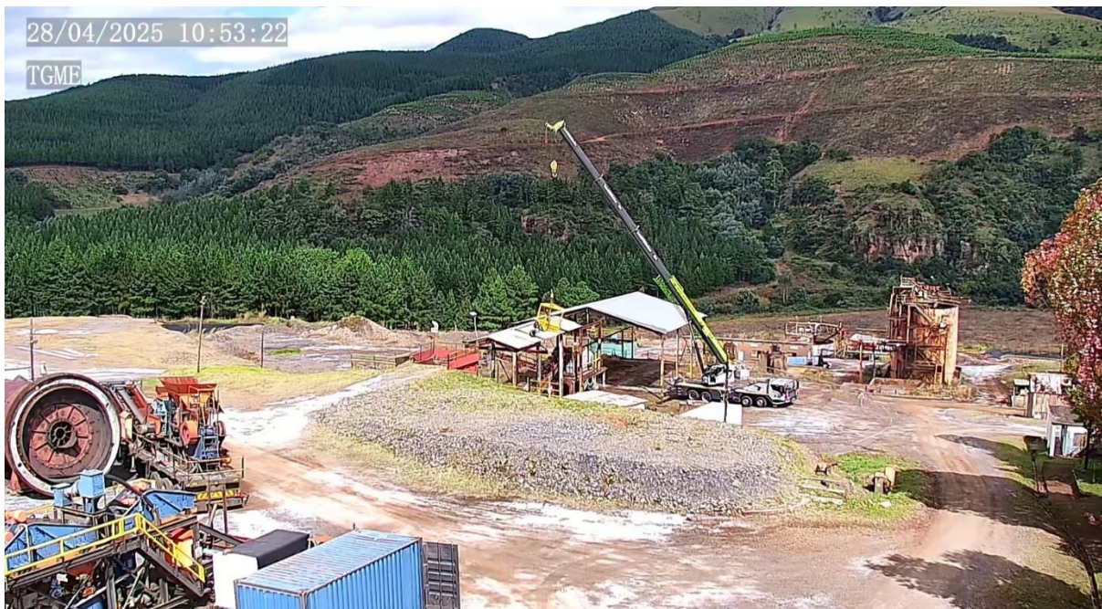
Figure 1: 50 Ton crane on site undertaking decommissioning activities
