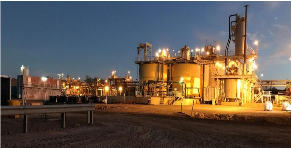
Figure A14: Existing CIL and Adsorption Tanks and Elution Column
