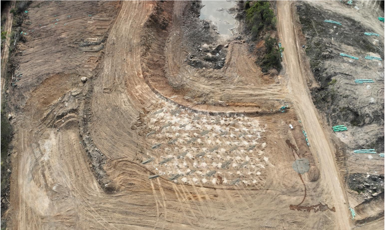
Figure 2: Aerial view of the Southern Starter Pit at Blackjack, with drill pattern completed and blast holes charged in preparation for first production blast.
