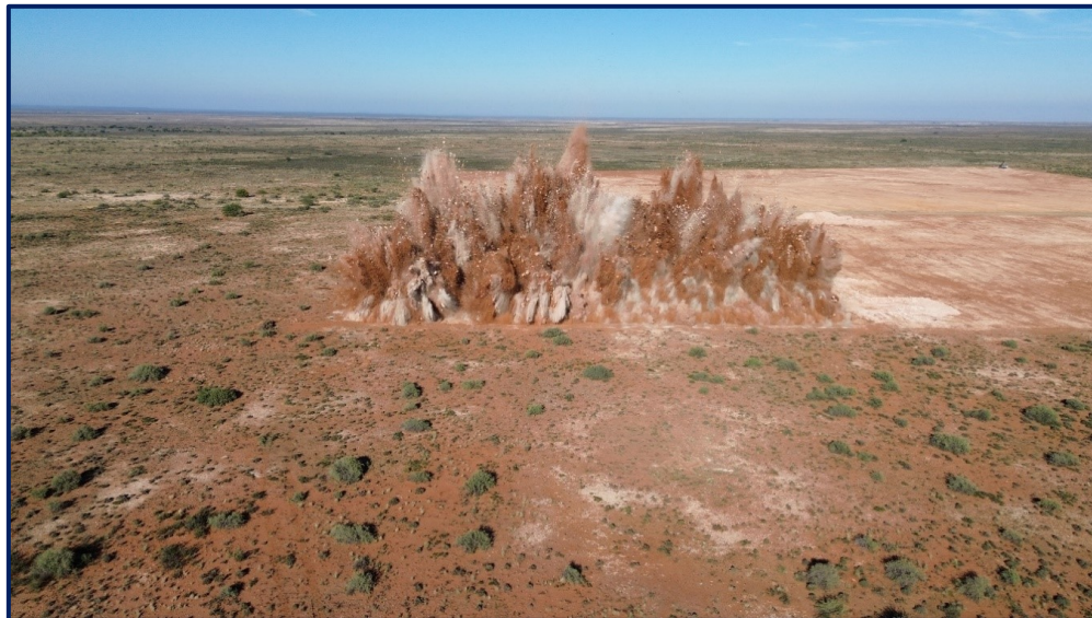
Photo 3: First Blast at 13ha Brine Water Storage Dam / TSF.
