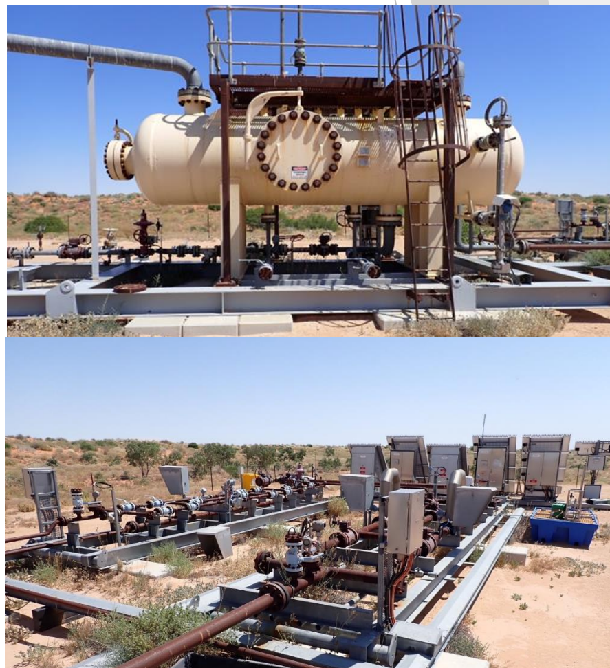
Figure 6: Gas/liquids separator in place at Vanessa facility
