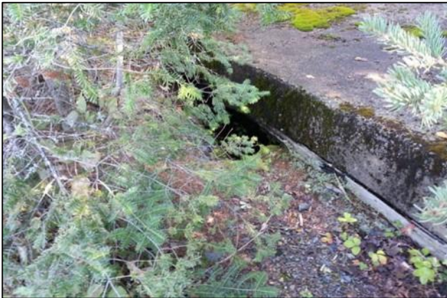
Concrete slab over entrance to mine shaft at Vanchester Prospect
