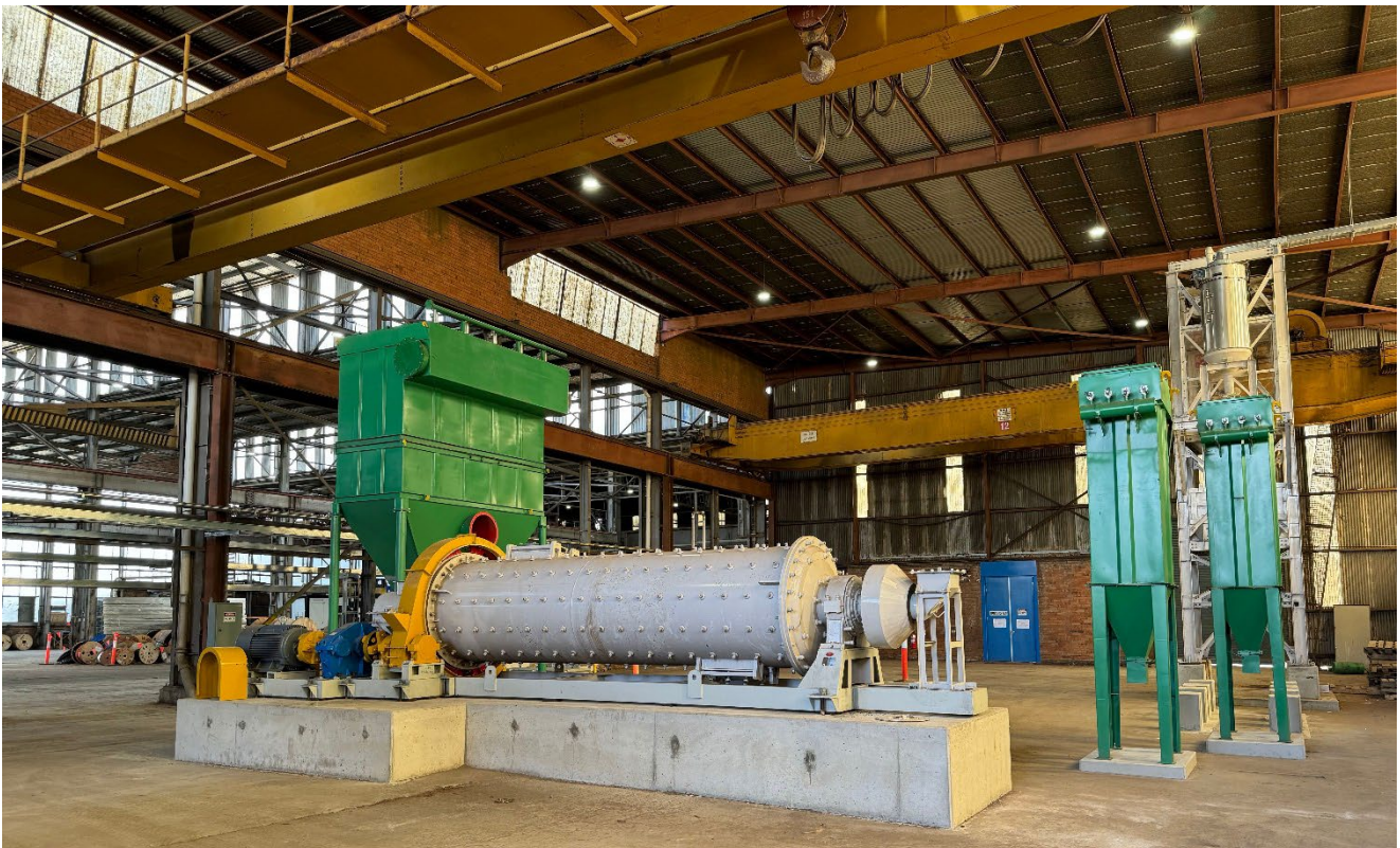
Figure: Briquette civil work completed with major equipment set in position on foundations
