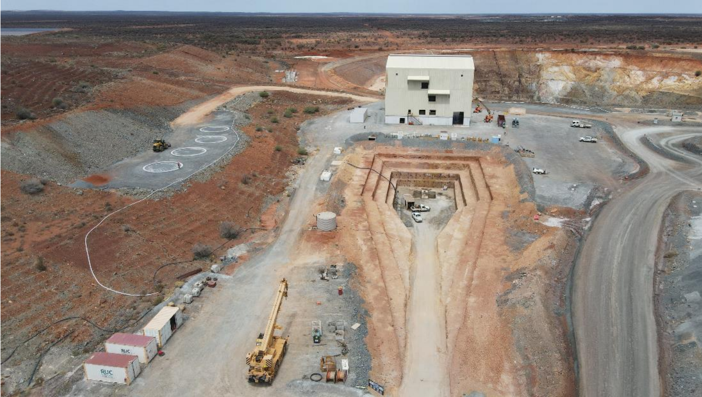
Winder house complete ready for winder installation
