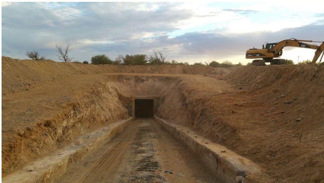
Figure 4: Fully exposed portal of decline roadway, which extends to 1200m below surface.
