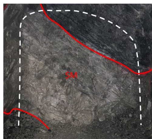
TBA 445 ore drive (4.5m W x 4.5m H) with a face grade of 8.8% Ni
