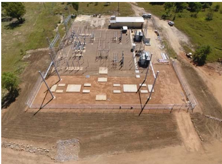
Figure 1: Ergon substation civil works complete.
