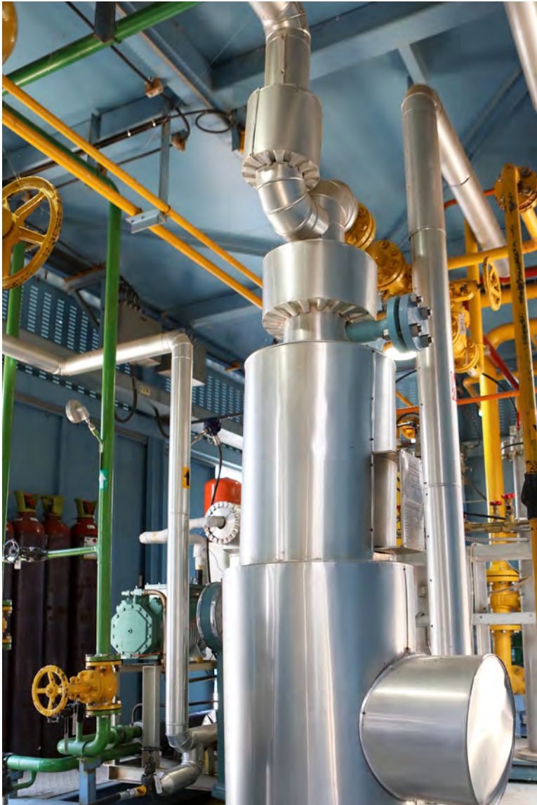
Mixed refrigerant loading manifold.
