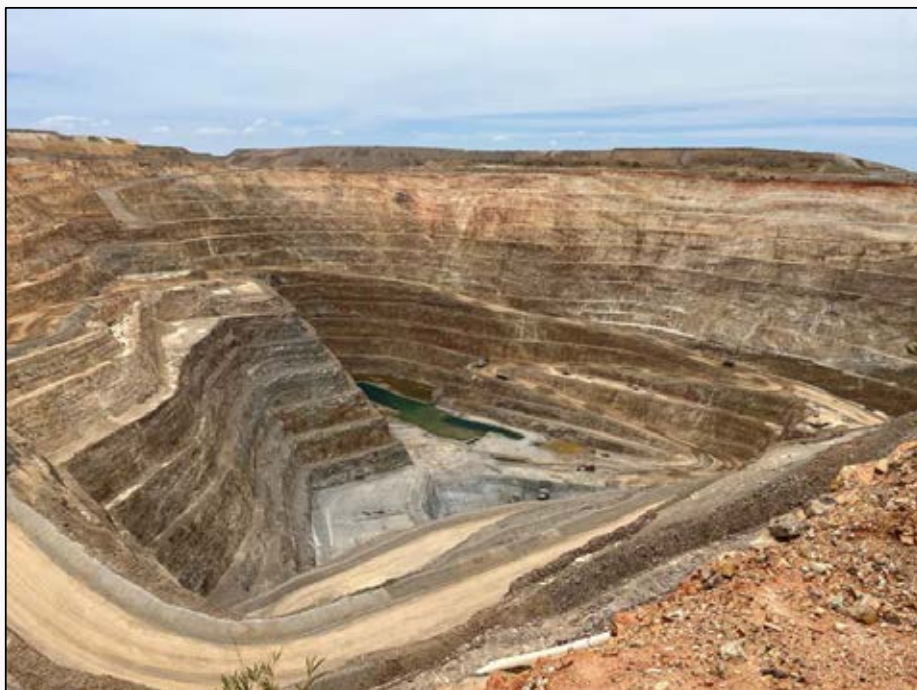
Figure 3-11: West Dome open pit (Stage 2 – flooded and Stage 8 – foreground)
