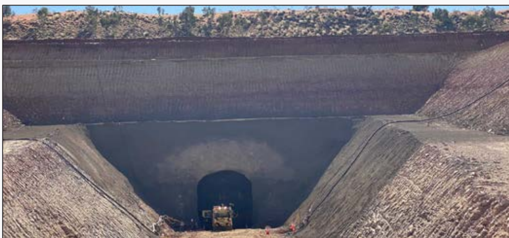
Figure 4-9: Early works (Stage 1) decline box-cut and portal
