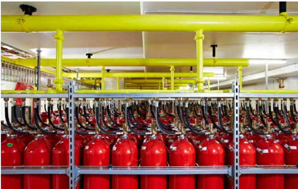
Inert gas fire suppression system
