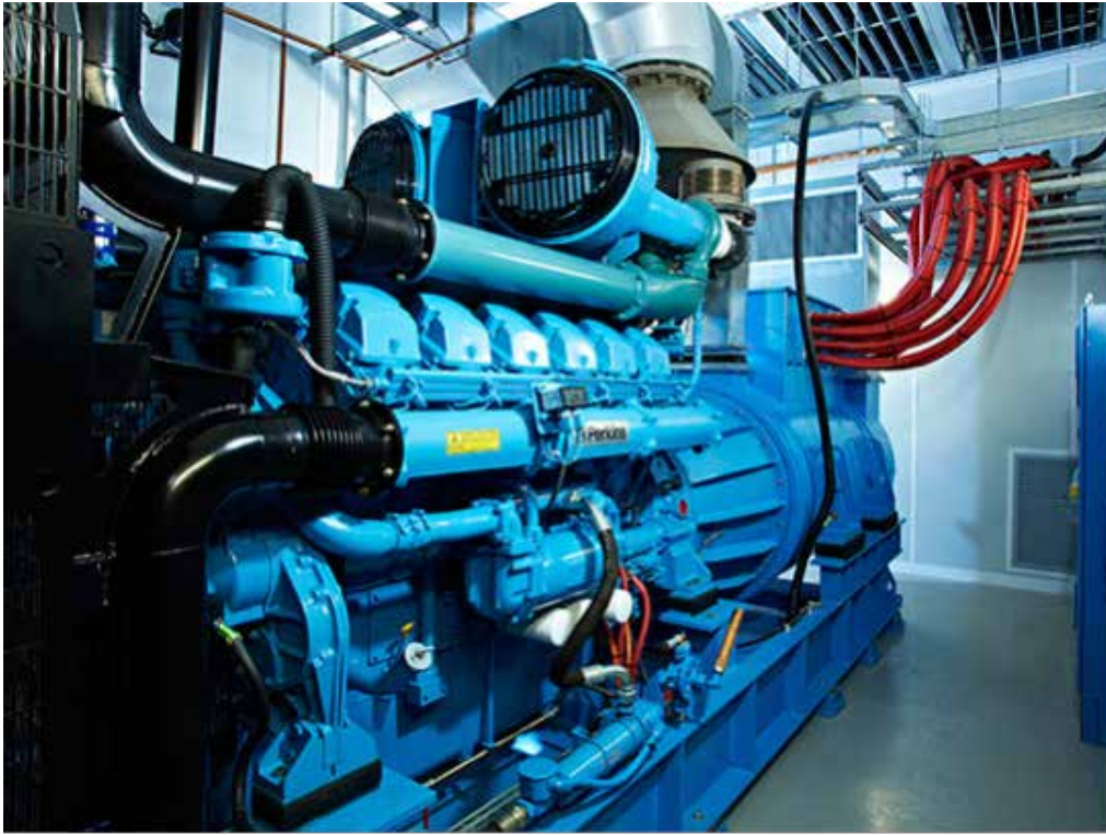
Perkins V12 diesel engine – part of a Pillar DRUPS unit
