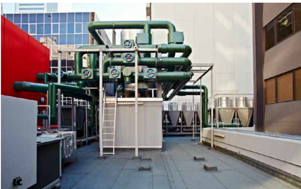
Air-cooled UNIFLAIR chillers (B1)
