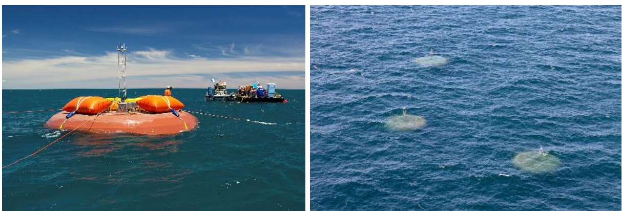
CETO 5 Unit 1 being installed in November, 2014 (L), CETO 5 three unit array operating (R)
