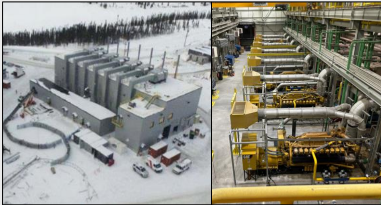
Figure 4. LNG-fired power station with a total capacity of circa 16MW
