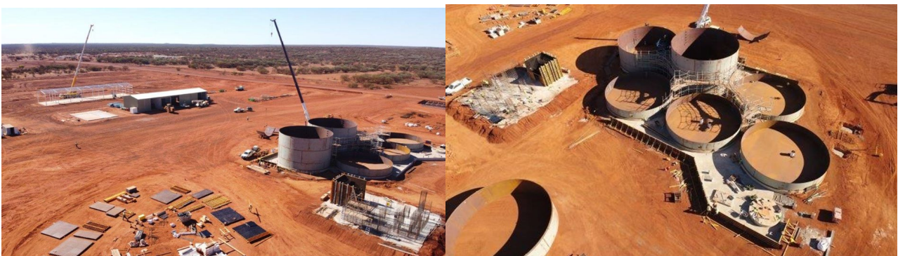
Figure 3: Processing plant construction progress and concrete foundations for the ball mill and CIL tank construction
