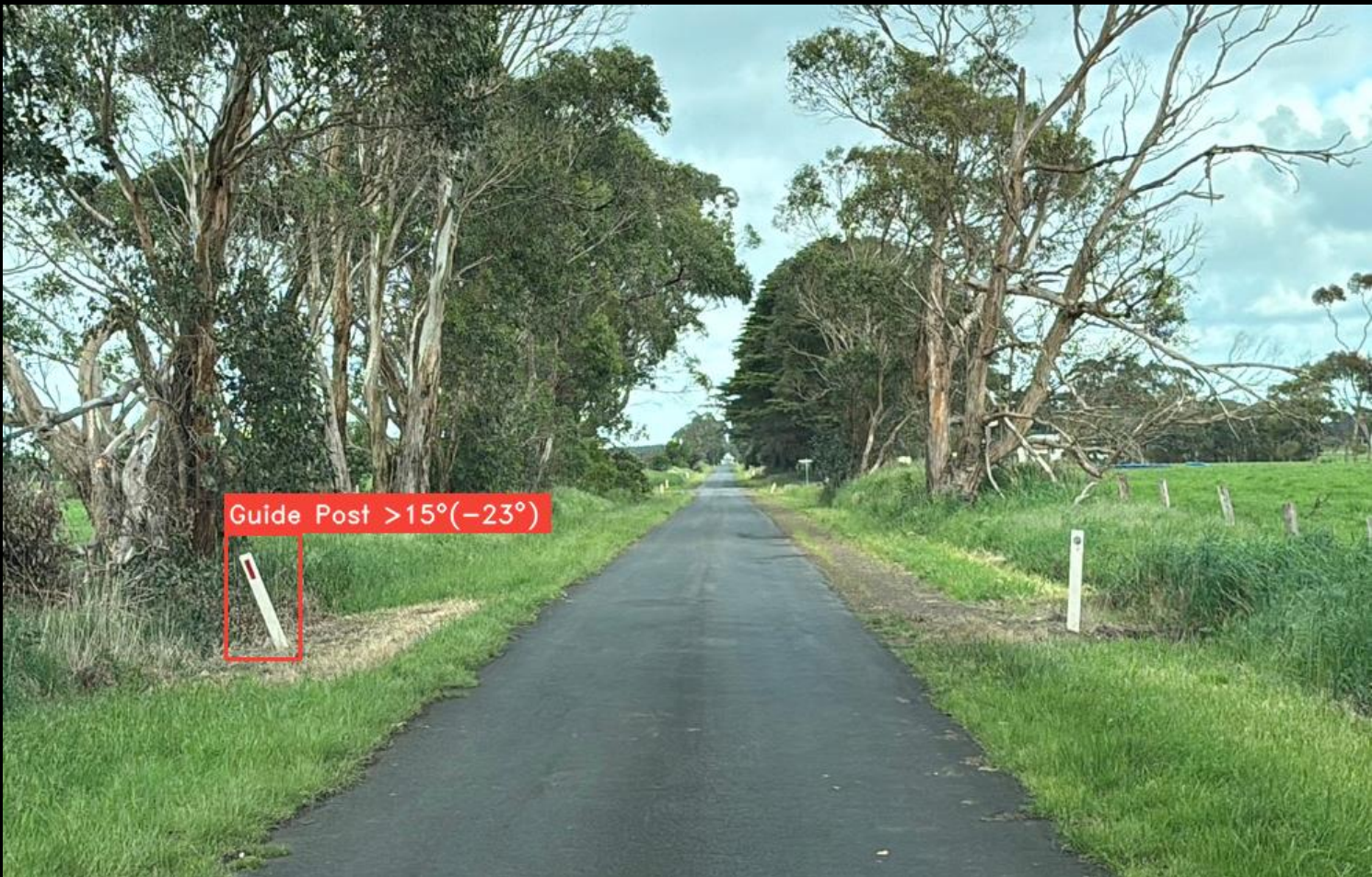
Detection for leaning guide post defects
