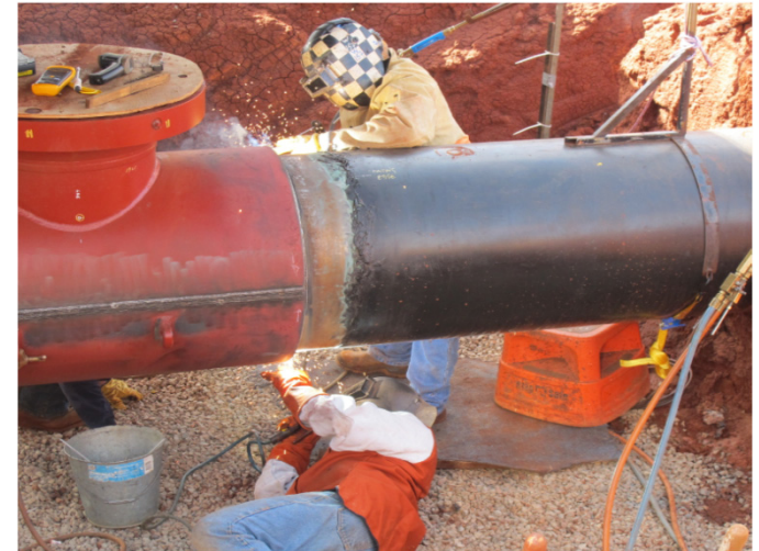
Pipeline welding work
