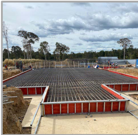
Figure Five | Primary Crusher Foundation Preparation
