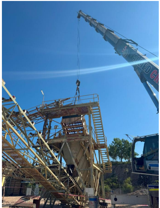
Lifting and Install New Shaker Screen
