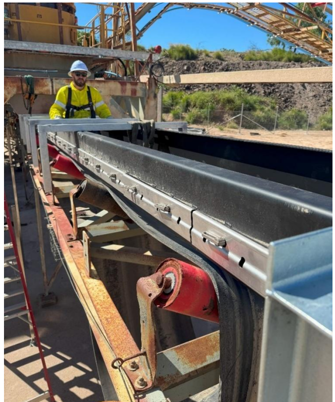
Installation of New Conveyor Skirting
