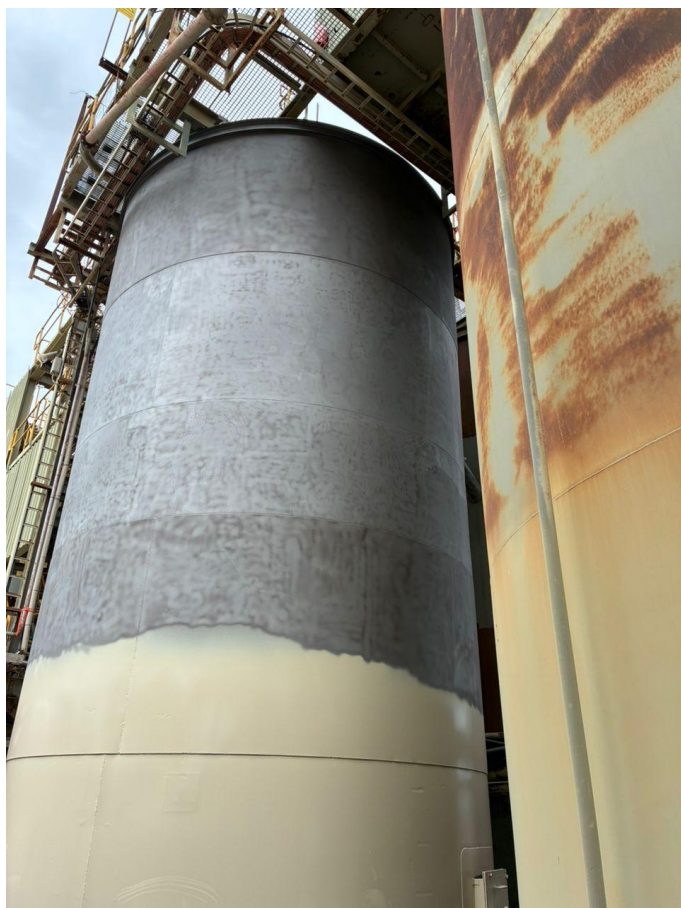
Commenced Blasting & Painting of CIL Tanks - 6 May 2025
