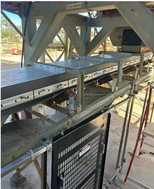
Installation of New Conveyor Skirting
