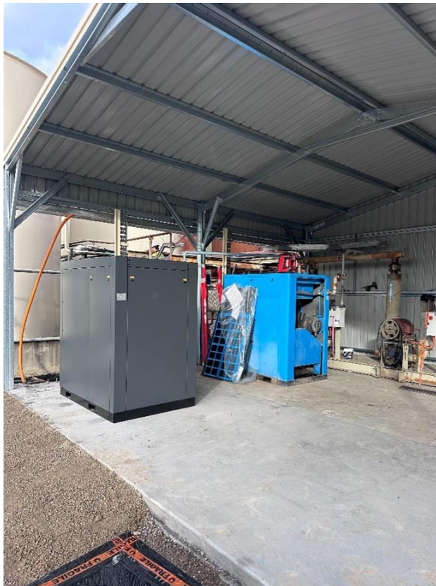
Installed New Air Compressor
